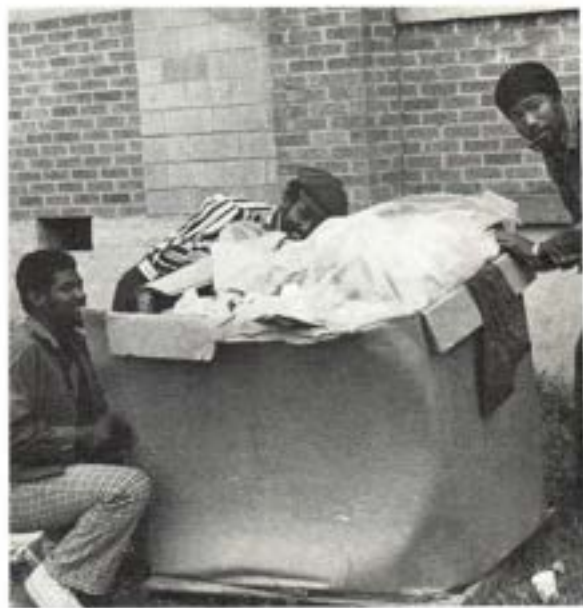
Three men finish a day's work on the Center.
