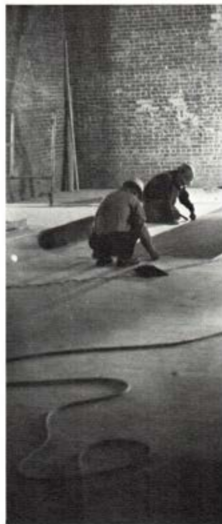
Workers put down flooring in the new auditorium.
