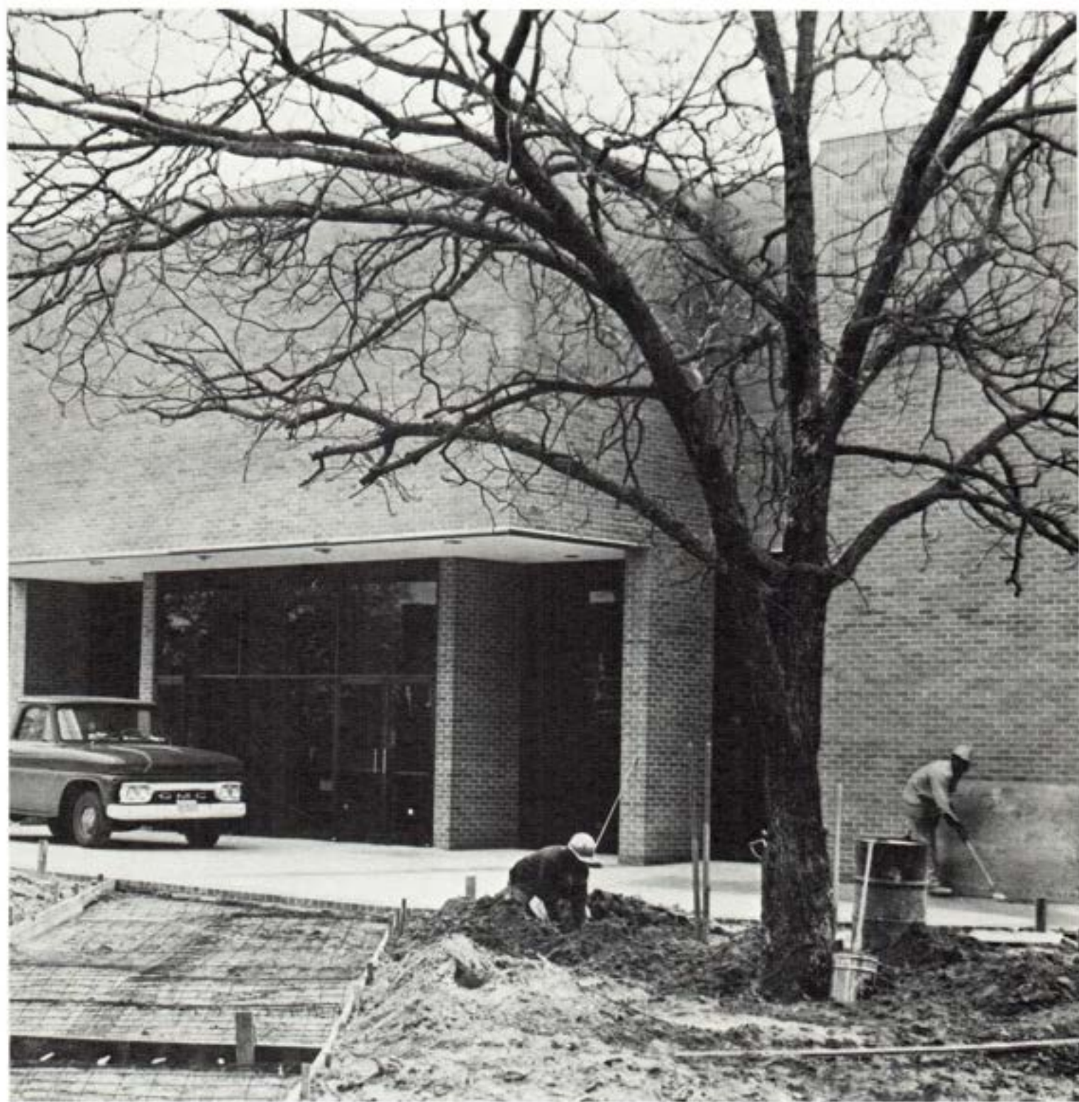
Workers lay sidewalks in front of the auditorium.
