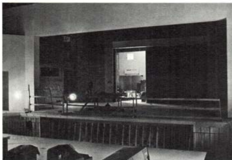
Harton Auditorium nears completion.
